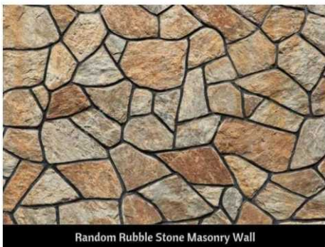
Random Rubble Stone Masonry Wall
