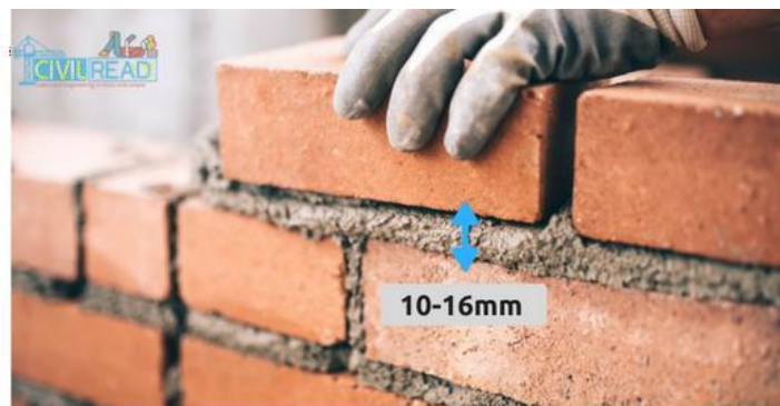
Mortar Thickness in Brickwork
