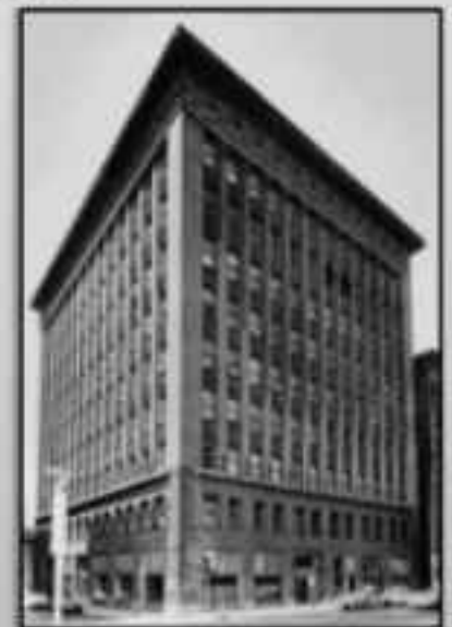
The Wainwright Building (1890)
