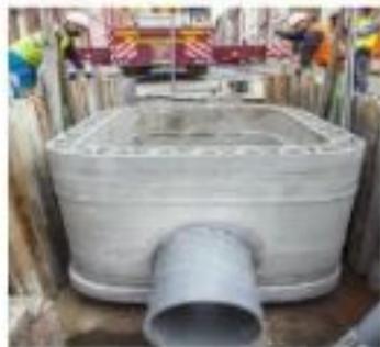
(b) 3D concrete printed storm drain
