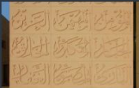
Al-Aziz Mosque Abu Dhabi, Light Transmitting Concrete Facade
