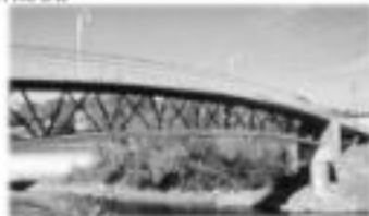
Figure 1: Bridge made of high performance concrete
